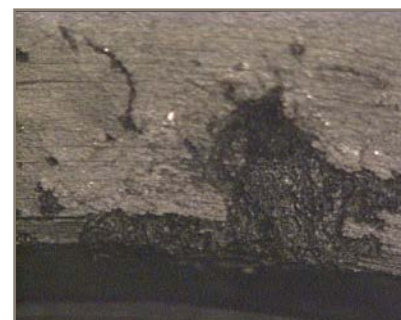
Pitting on filter end-cap
